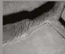
Cracking Between Tread
